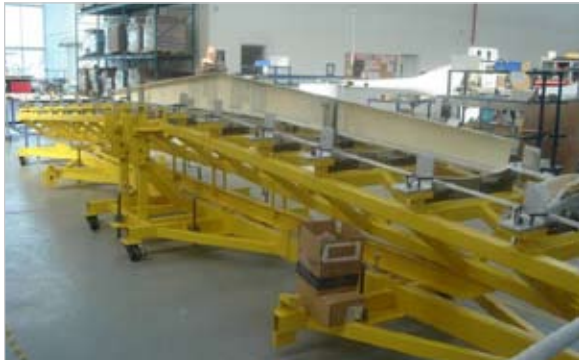
Fixturing the main Spar is the first step in the wing structure assembly.
